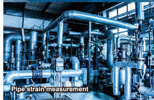
Brake and pipe strain measurement
